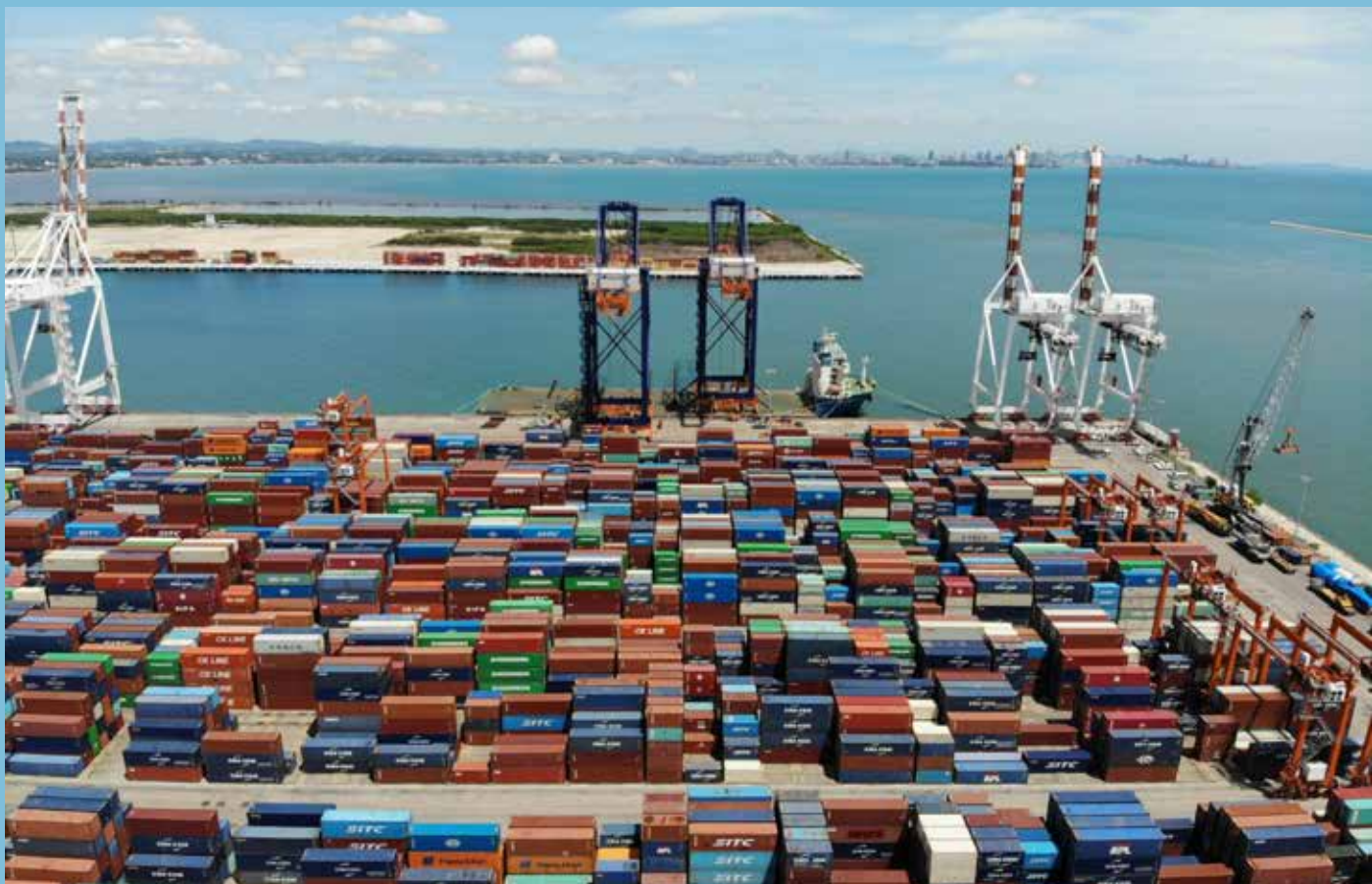
LCIT's C3 Terminal at Laem Chabang Port, Thailand
